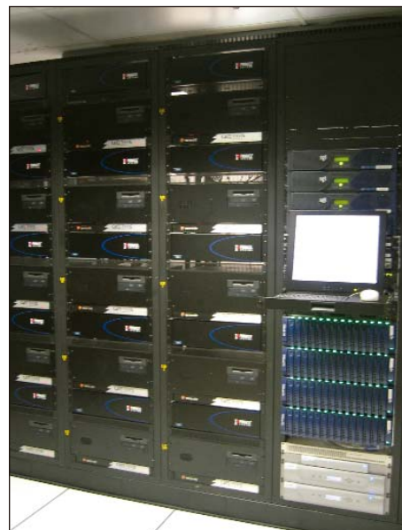
An NBA Entertainment server facility
